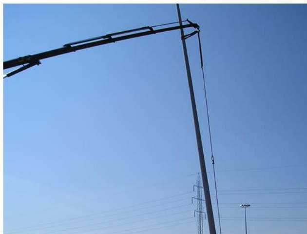
4. Mast i lodret position over fundament.
